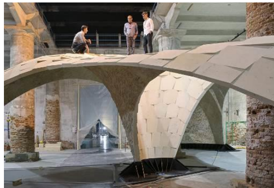
Fig. 5. Brick Vault in the display [2].
